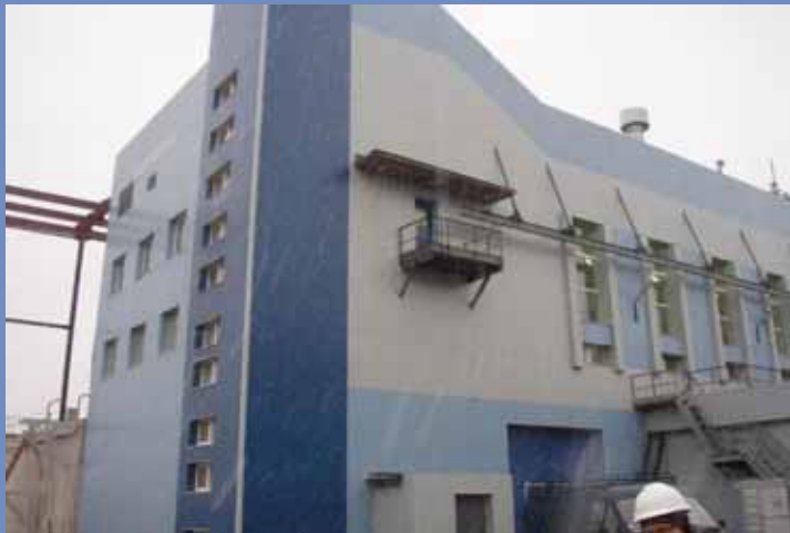
Northern and SW Incinerators in 2007
