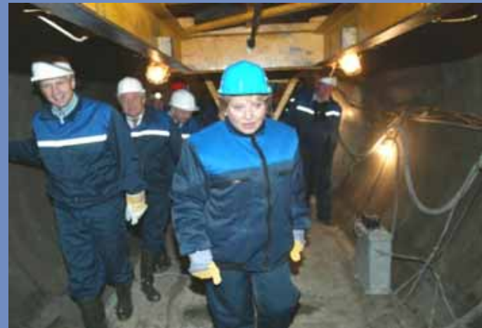
Northern Tunnel Collector project now under construction
